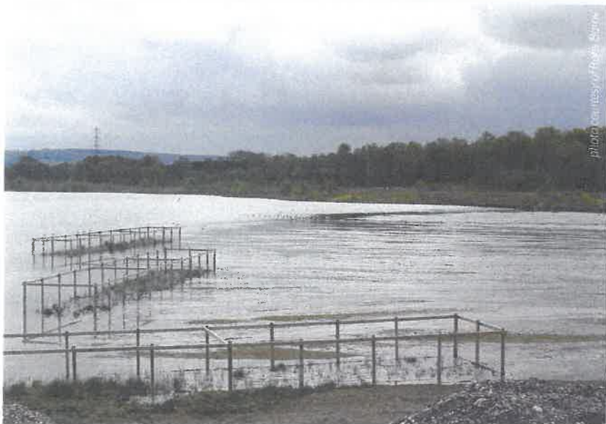
Figure 1: silt reed restoration in progress
